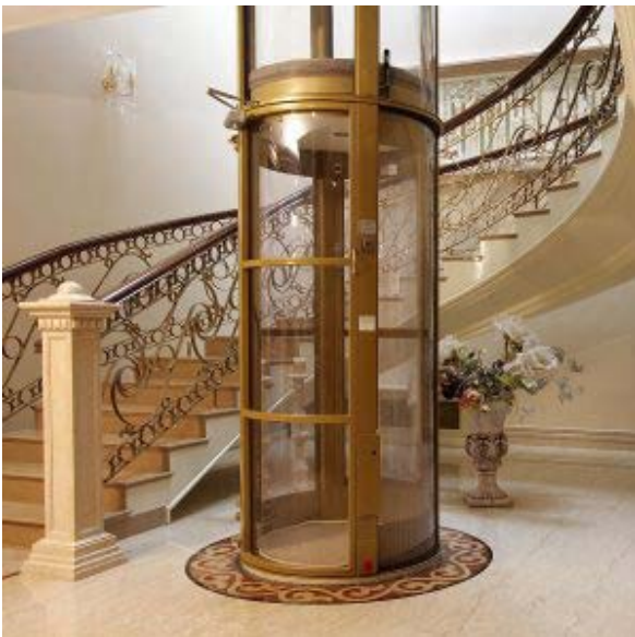
Figure 2. Pneumatic Elevator
